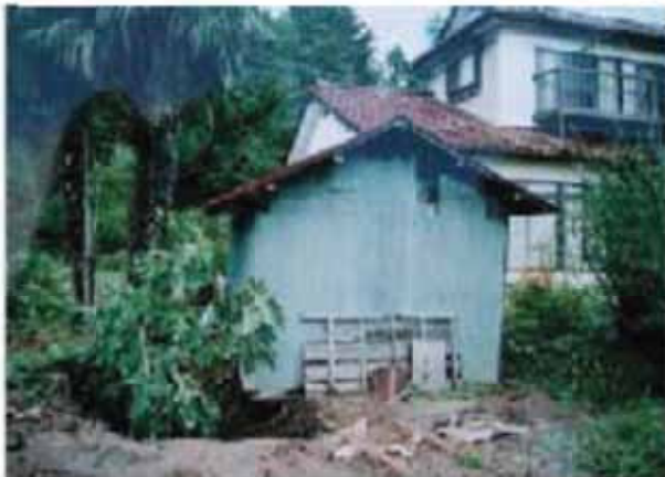
(b) 陥没穴と噴砂
